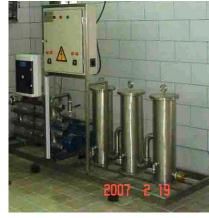
Stainless Steel chase which mounted UV+ Buster pump+ Micro filters & Control box
